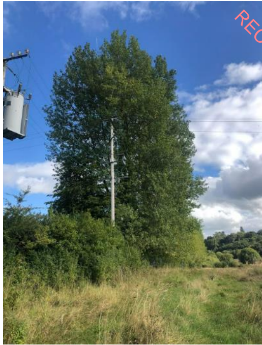
[Photo 19; Poplars view looking south east.]
