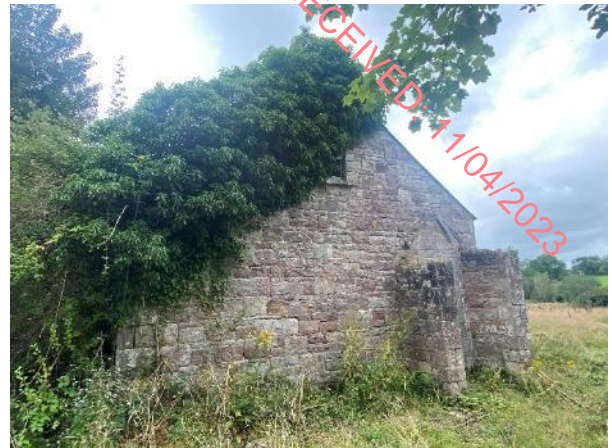
A8. Eastern elevation of B4 showing dense ivy and access point.
