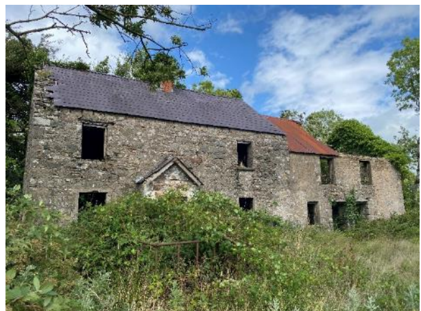
A6. Southern elevation of B2.
