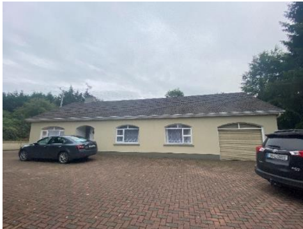
A1. Eastern elevation of B3.
